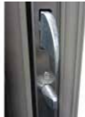
Multipoint 3 hook lock to opening door
